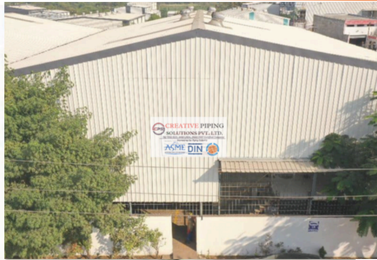
Creative piping (UNIT II)
