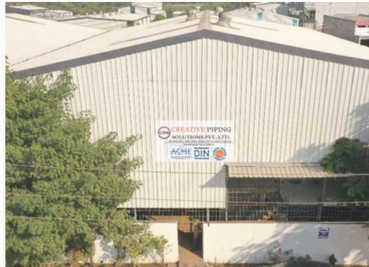
Creative piping (UNIT II)
